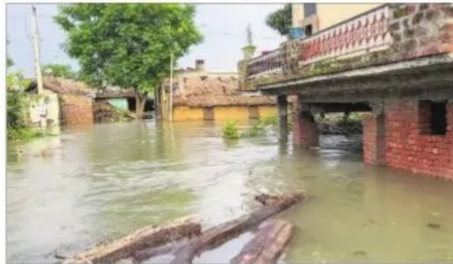
Houses submerged in floodwater at Bhanam village in Ropar, ANI
